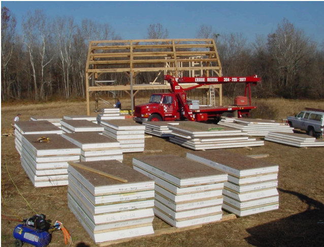
IMAGE 5.6: SIPS STAGED ON JOBSITE
